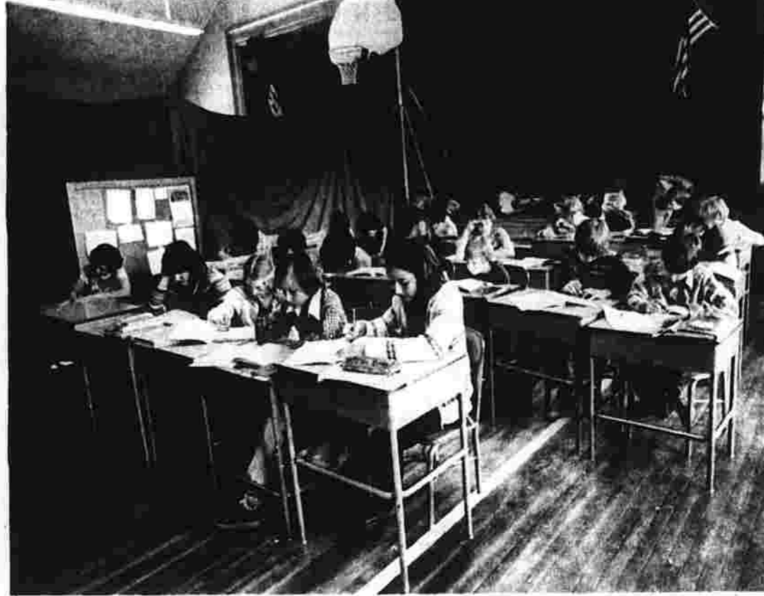
Bentley renovation begins
